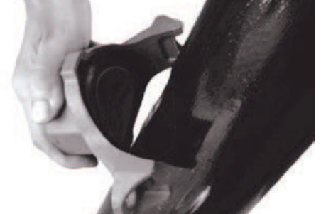
3. Gasket installation
