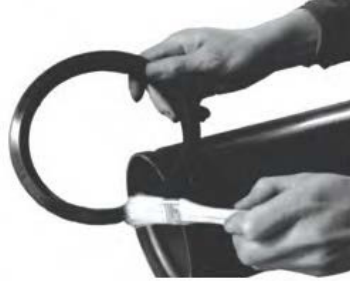
2. Lubricate Gasket
